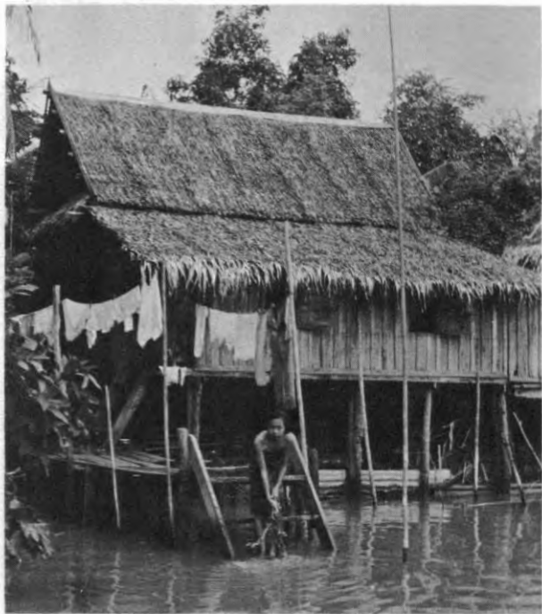
Fronting a "klong," this rural home is built on stilts.
